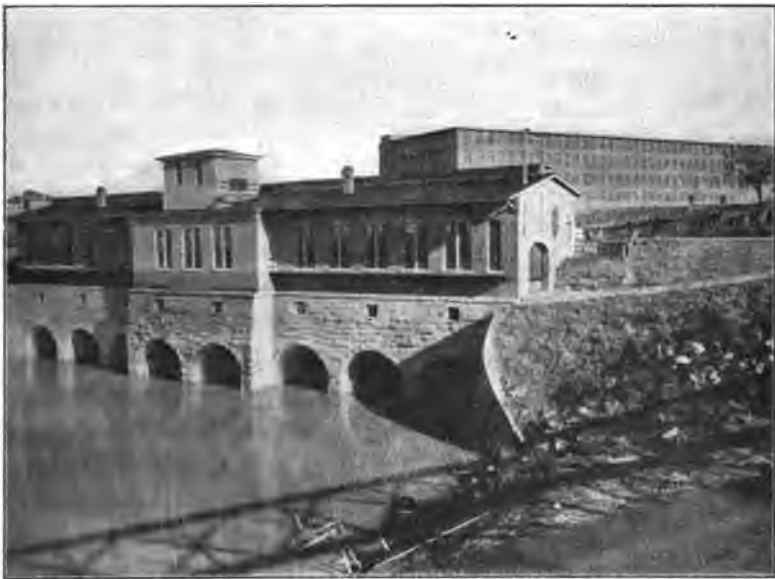
POWER PLANT, COLUMBIA, S. C.—10,000 H. P. DEVELOPED FROM COLUMBIA CANAL.
